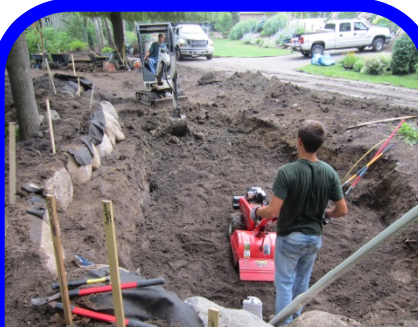
Loosening of soils at the bottom of bioretention cell prior to engineered soil placement
