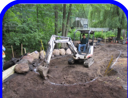
Excavation of bioretention cell with tracked excavator
