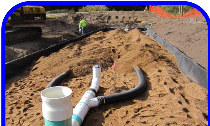
Perforated underdrains with a flow controlling valve were installed and covered with an 18 inch depth of iron enhanced sand filter material.
