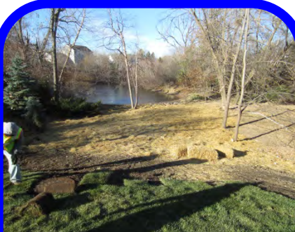
Installation of sod and mulch with seed to vegetate soils after installation of pipe.
