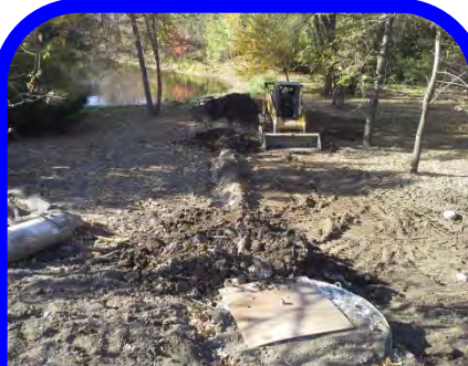
Installation of pipe to redirect runoff from 6.2 acres into wet sedimentation pond.
