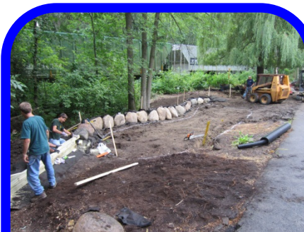
Installation of boulder retaining wall and wood weir to control outlet elevation
