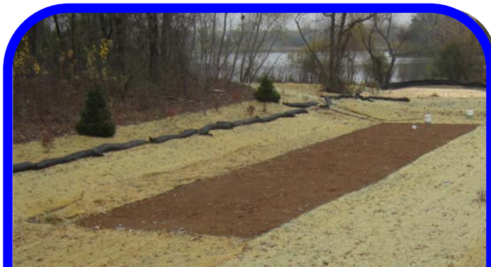
A native seed mix was covered by erosion control blanket and highlighted with shrub plantings. The cells will remain off-line until 2014 to allow the native seed to establish.
