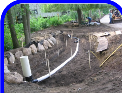
Installation of underdrain, valve, and engineered soils
