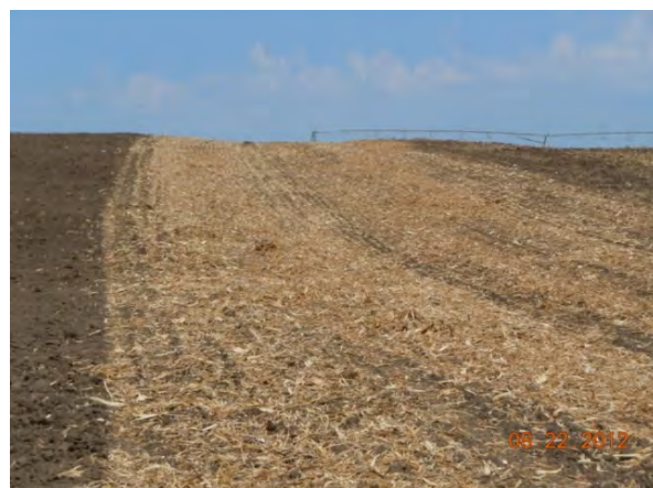
Re-established grassed waterway, looking north, after straw has been crimped within the channel.
