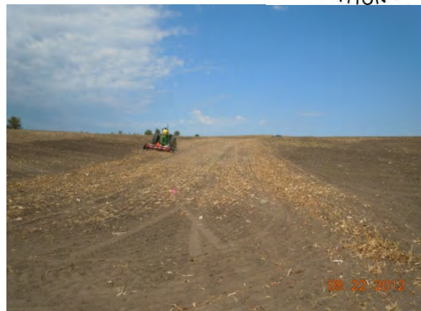
Re-established grassed waterway, looking north. Landowner is crimping straw into the soil to stabilize the channel until grass is established.
