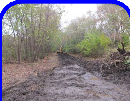
Removal of clay layer to expose underlying sandy soils in the infiltration basin
