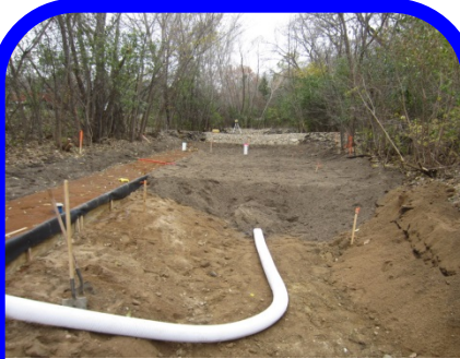
Installation of iron-enhanced sand filter, engineered soils, and underdrain system
