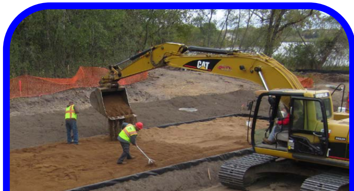
The iron sand mixture in the filtration area contained 5% iron filings by weight. The infiltration areas outside of the forms contained 70% coarse washed sand, 15% compost and 15% sphagnum peat.
