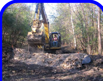
Installation of rock weepers for pretreatment to remove sediment upstream of infiltration basin
