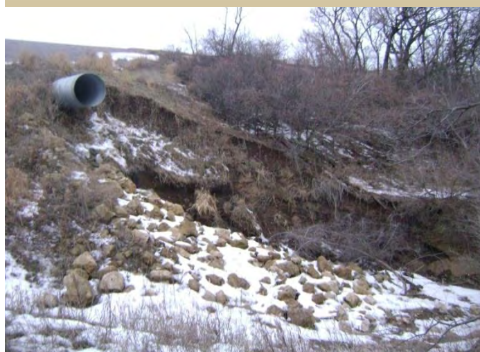
Runoff from the pipe shown in this photo carved a ravine that allowed sediment to flow into the Mississippi River.
