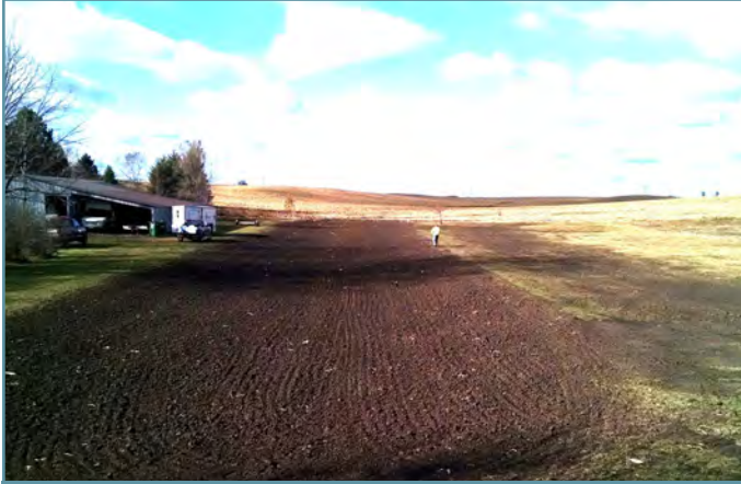
Final graded grassed waterway during seeding, looking west
