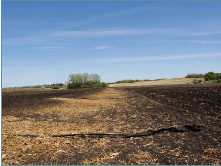
Grassed waterway after seeding, mulching and installation of fabric barriers across waterway.
