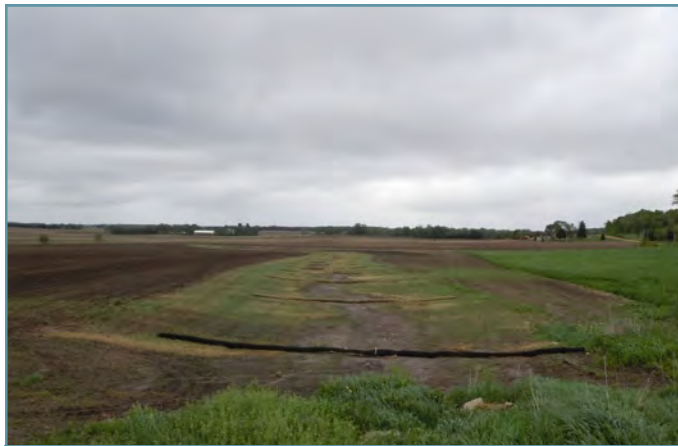
Straw wattles have been installed to control erosion and vegetation is starting to grow
