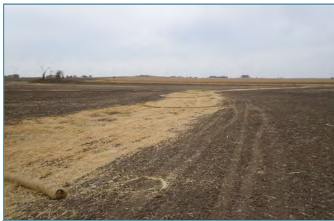
Waterway #3, After the waterway was seeded, mulched and straw wattles were installed.
