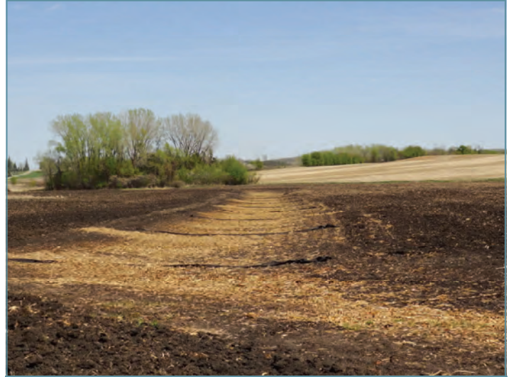
The fabric barriers serve as temporary check dams until grass is fully established.
