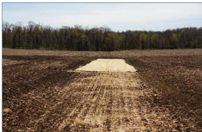
Erosion blanket, fabric barriers, and crimped straw. Three forms of protection on the recently graded waterway.
