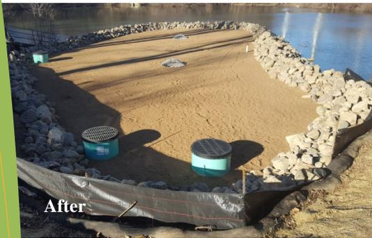
This iron-enhanced sand filter incorporates sand mixed with iron. The iron removes dissolved phosphorus from stormwater while the sand removes particulate-bound phosphorus, helping to improve nutrient impaired waters.
