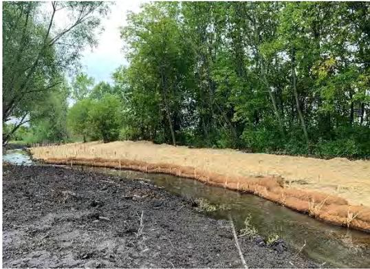
Stream restoration included installing numerous in-stream habitat features, narrowing portions of the channel that are over-widened, stabilizing the bank, and improving riparian conditions to limit sedimentation and improve wildlife habitat.
