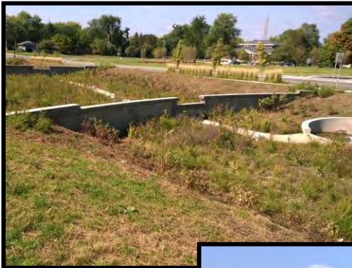
"Stepped" infiltration basin in Oakdale, MN.
