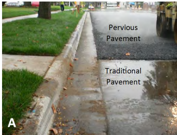
Images of pervious pavement in a parking lot (A) and low traffic areas (B).
