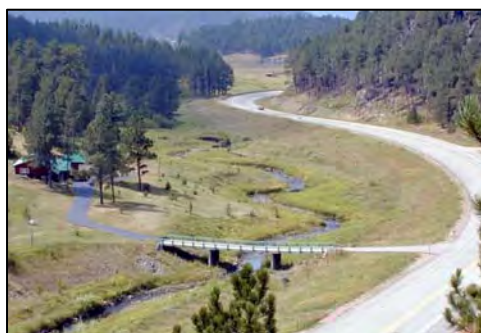
Figure B-6. This segment of Spring Creek in the Black Hills was relocated and restored as part of new highway construction (photo Inter-Fluve).
