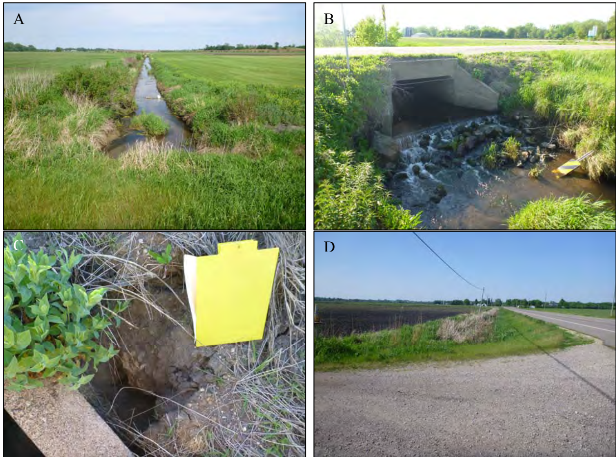
Figure C-12, Tributary 2, 2A: A) Tributary 2 looking downstream from Blaine Ave. B) looking upstream at perched culvert under Clayton Ave. C) hole developed between culvert and road at Clayton Ave. D) Tributary 2A looking downstream along Blaine Ave.
