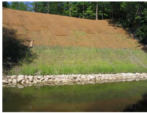
Figure B-4: Rock toe, stacked geocells, and fabric at hart Park, Milwaukee.
