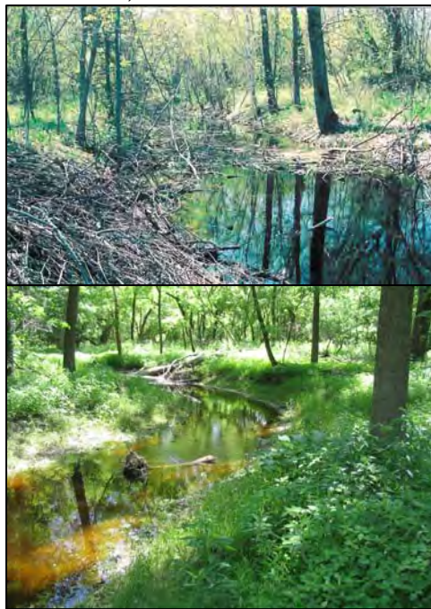
Figure B-7. This segment of Trout Creek on the Oneida Reservation was channelized in the early 1900s (top). The restored segment (bottom) shows floodplain excavation, woody debris habitat installation and native plantings (photo Inter-Fluve).
