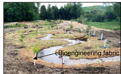
Figure B-3: Grasses are beginning to grow through biodegradable bioengineering fabric along this restored stream (photograph: Inter-Fluve).
