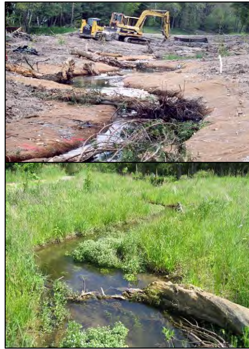
Figure B-8: Stream restoration in agricultural areas can sometimes involve reconstructing a new valley form or incipient floodplain (photograph: Inter-Fluve).
