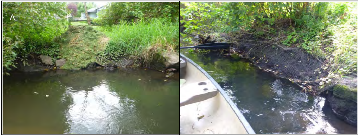
Figure C-10, Reach 9: A) Taken at Station 63,450. B) Looking at right bank at Station 63.350 to show bioengineering restoration techniques, including root wad placement, bioengineering fabric, and rock toe protection.
