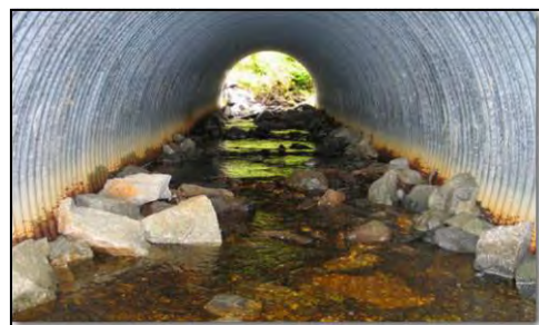
Figure B-2: Bottomless arch that is partially buried for better habitat and fish passage conditions.
