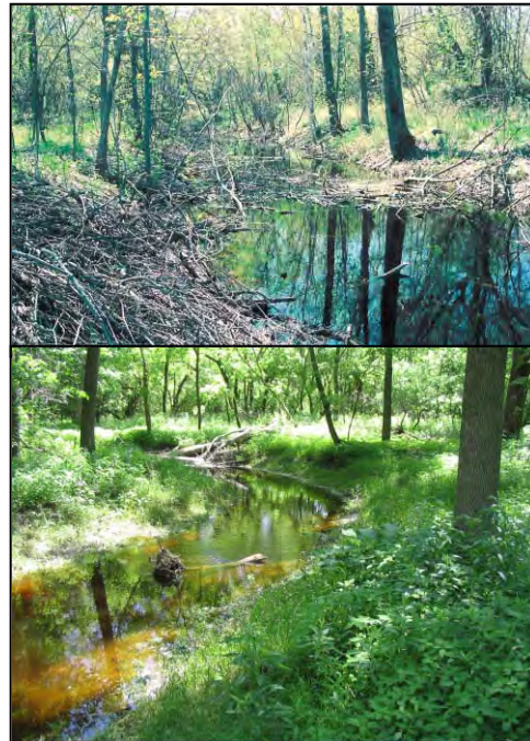
Figure B-7. This segment of Trout Creek on the Oneida Reservation was channelized in the early 1900s (top). The restored segment (bottom) involved floodplain excavation, woody debris habitat installation and native plantings (photo Inter-Fluve).
