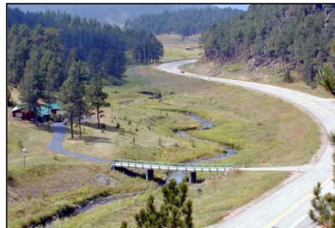
Figure B-6. This segment of Spring Creek in the Black Hills was relocated and restored as part of new highway construction (photo Inter-Fluve).
