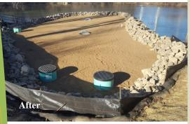
This iron-enhanced sand filter incorporate sand mixed with iron. The iron removes dissolved phosphorus from stormwater while the sand removes particulate-bound phosphorus, helping to improve nutrient impaired waters.
