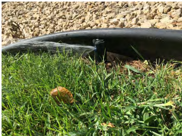
Figure 19 (below): Rotor unable to pop up due to landscaping
