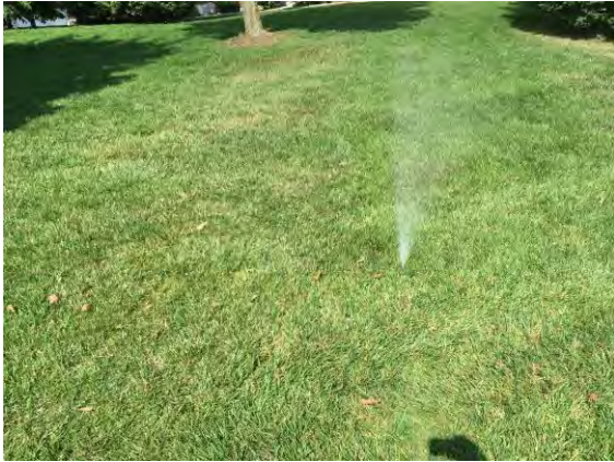
Figure 20 (above): Rotor not rotating, dry areas beginning to appear
