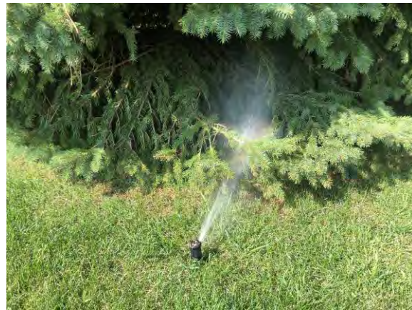
Figure 20 (above): Rotor not rotating, dry areas beginning to appear
