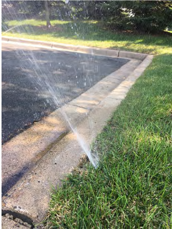
Figure 12 (above): Rotor spraying onto pavement
