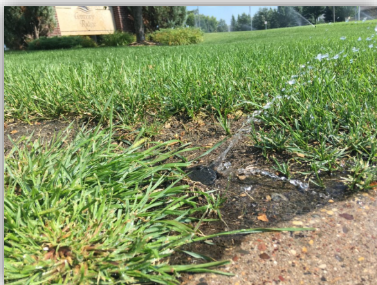
A broken sprinkler head can waste thousands of gallons of water per week.
