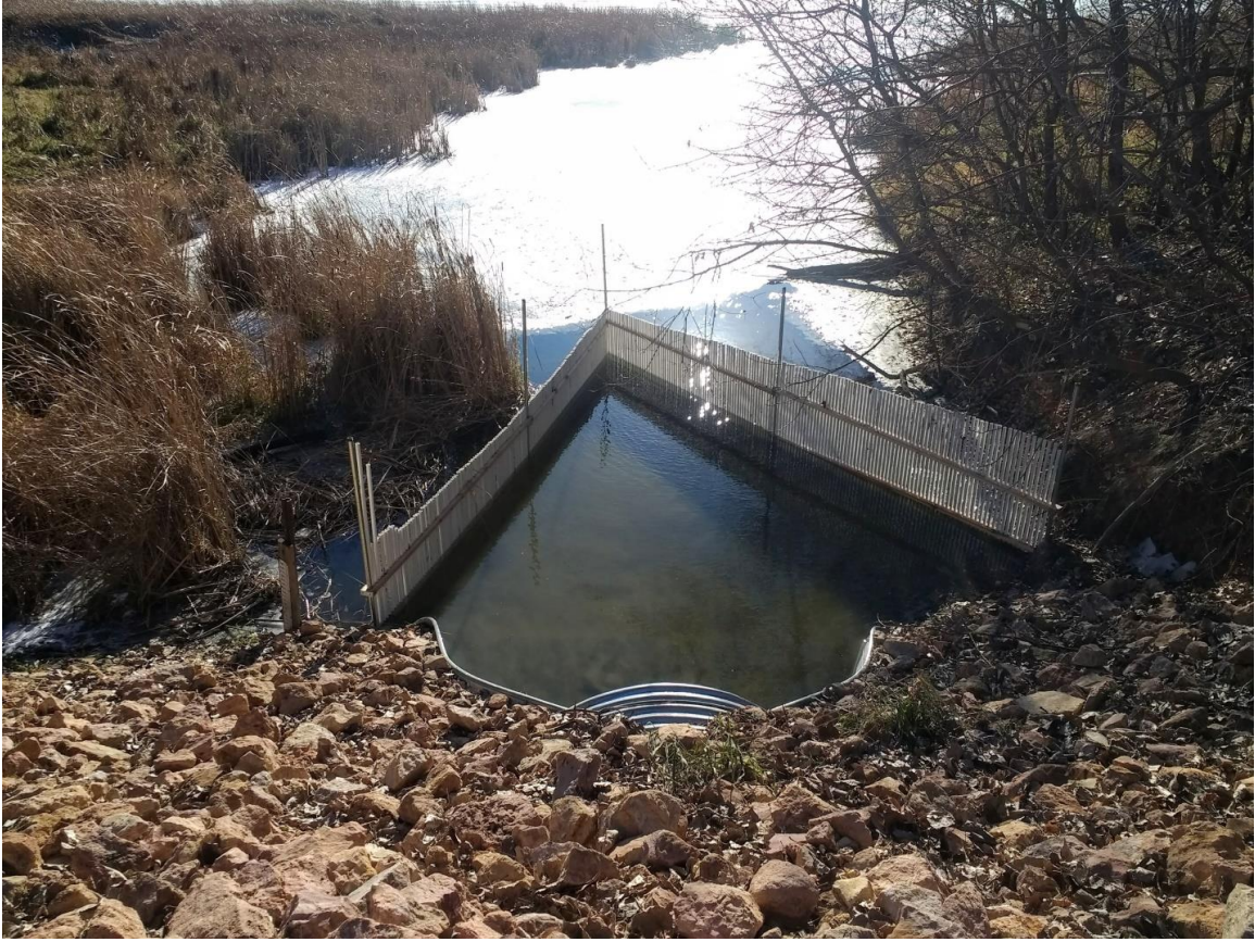
Figure 6: PVC semi-permanent fish barrier example.
