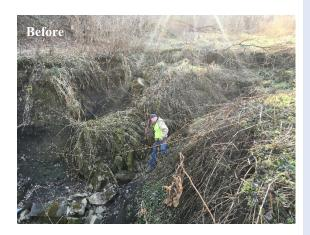
Stabilizing waterways and ravines with deep erosion prevents soil from moving downstream and causing sedimentation and negative water quality impacts. Stopping continued erosion also prevents migration of the ravine upstream, protecting infrastructure.
