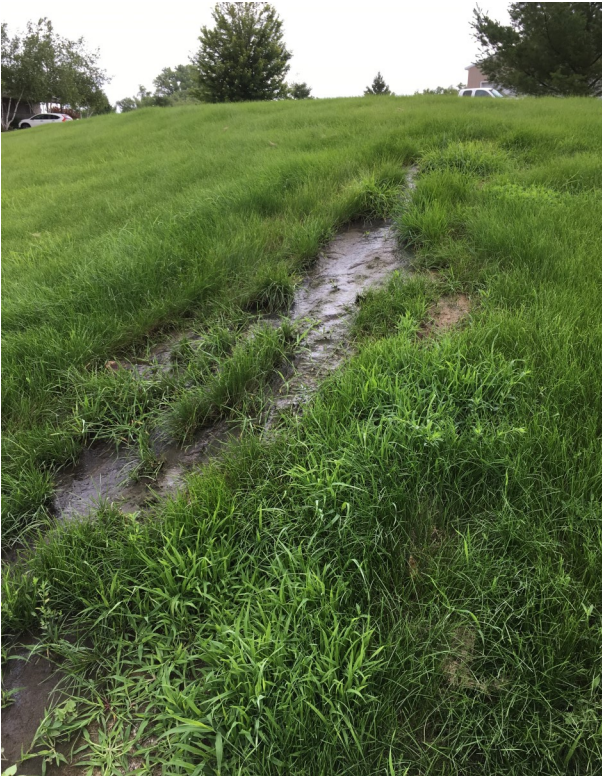
Failing wastewater drainfield
