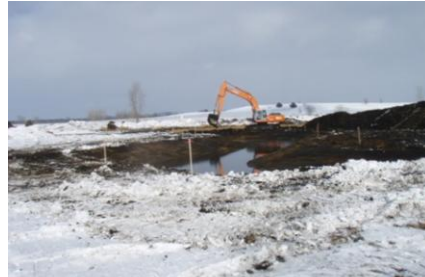
Winter construction of stream meanders
