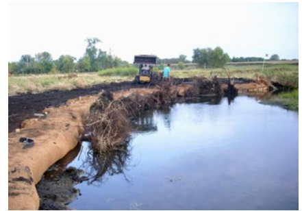
Coarse wood toe will prevent streambank erosion
