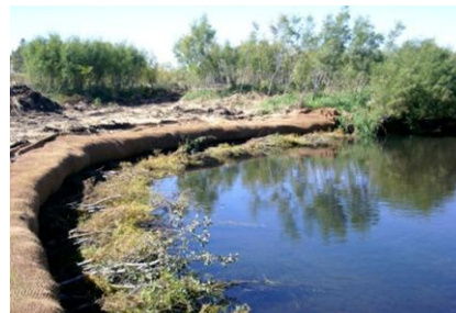
Coarse wood toe will prevent streambank erosion
