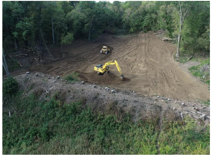
Figure 3. Eastern basin during the sediment cleanout process.
