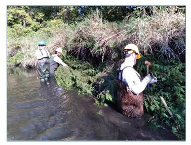
Crews harvested cedar trees and anchored the trees along eroding portions of the streambank in a practice called cedar tree revetment. This practice will help reduce future erosion and stabilize the eroding banks.
