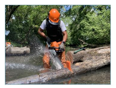
Smaller branches were removed by hand. Larger logs were cut into manageable sizes using chainsaws and then removed from the river channel.
