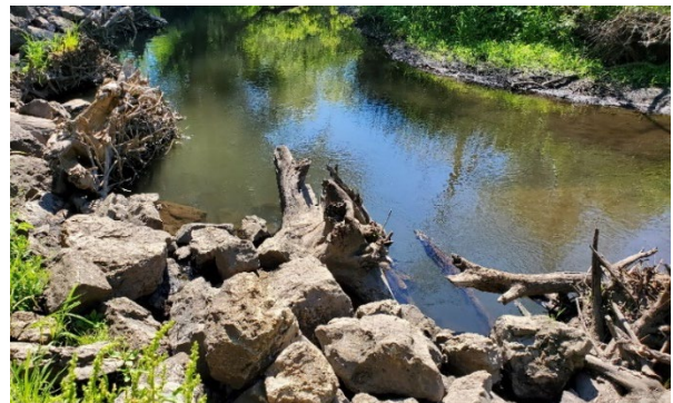
The bank of the Vermillion River in Rambling River Park, showing the cedar tree revetments and rocks.
