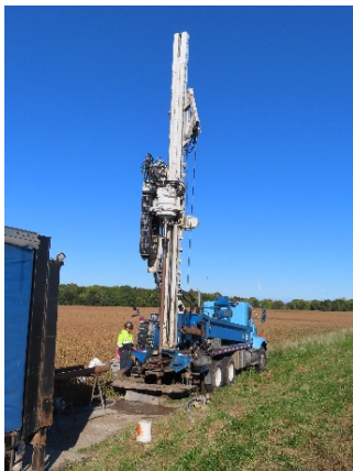
Shallow monitoring well being drilled. A new water monitoring network provides improved water quality data.
