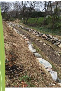
Phase 2 of the channel stabilization reduced 30 tons of sediment and 6 pounds of phosphorus from reaching Lake Marion annually.
