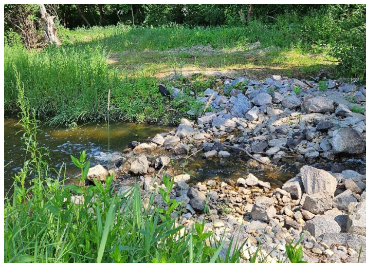
Figure 3. North Creek with rock checks installed.
