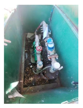
4" municipal water supply into 1.5" meter and Wilkins 975backflow prevention assembly tested 6/9/22.
