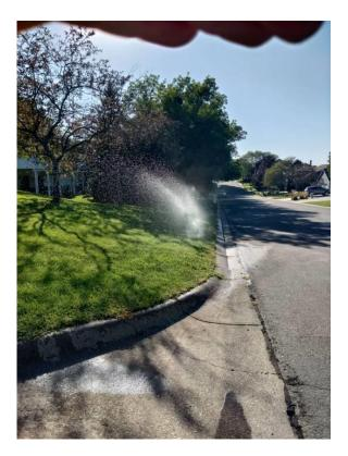
Sta 8 - 18-20 PgP & Rain Bird 5004 sprinklers mixed along Hyland Point Ct. Most PgP sprinklers have leaking seals & lots of runoff after a few minutes of operation.
