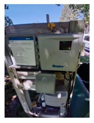
Hunter Pro -HC SMART-ready controller. Irritrol basic wireless rain sensor, not connected.
