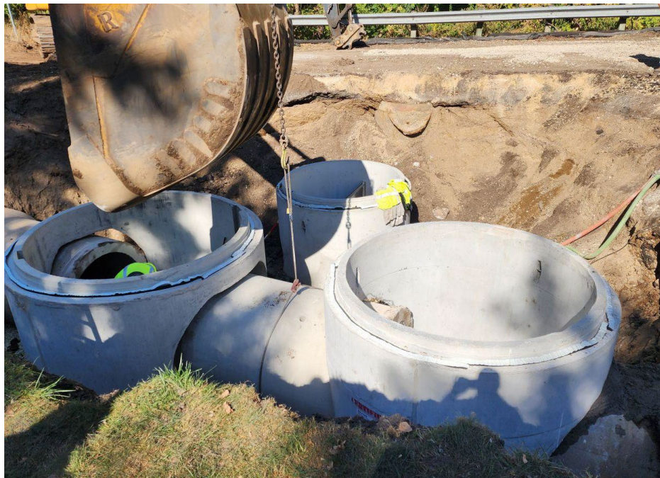
Figure 2. An example of a hydrodynamic separator being installed.
