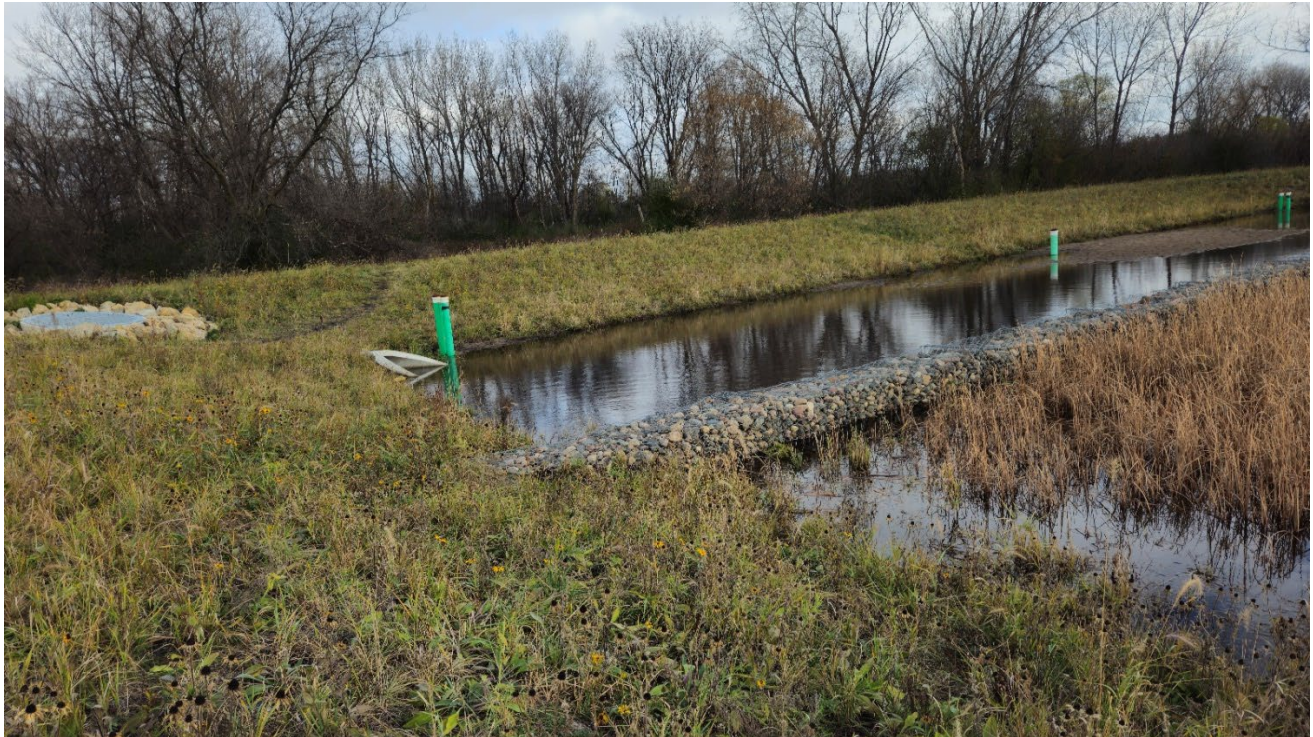
Figure 1. The completed dry pond and wet sedimentation forebay with rock gabion wall, November 2024.
