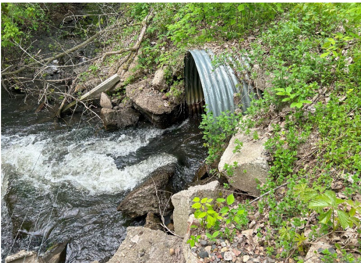
Figure 2. Downstream end of the pipe culvert slated for replacement at the field road.
