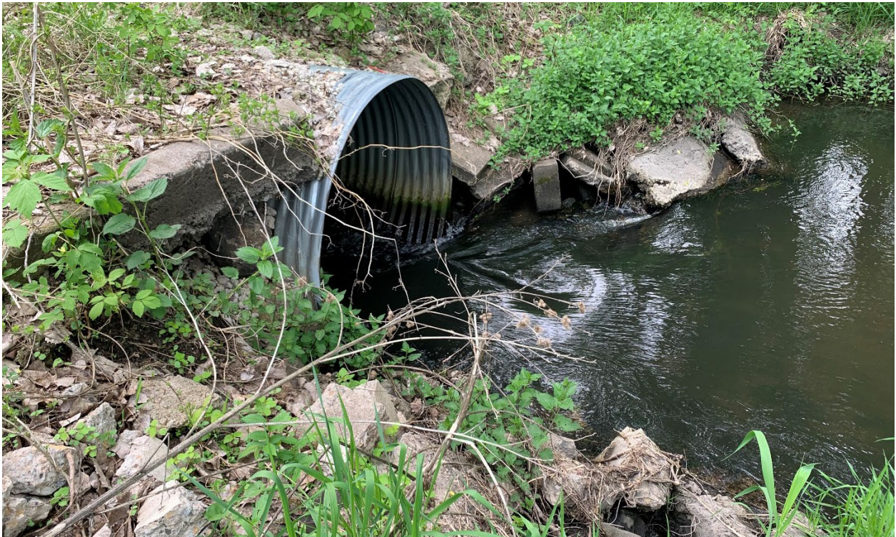
Figure 1. Upstream end of the field access road culvert on North Creek slated for replacement. The photo demonstrates the sharp acceleration of the stream velocity as it enters the culvert.
