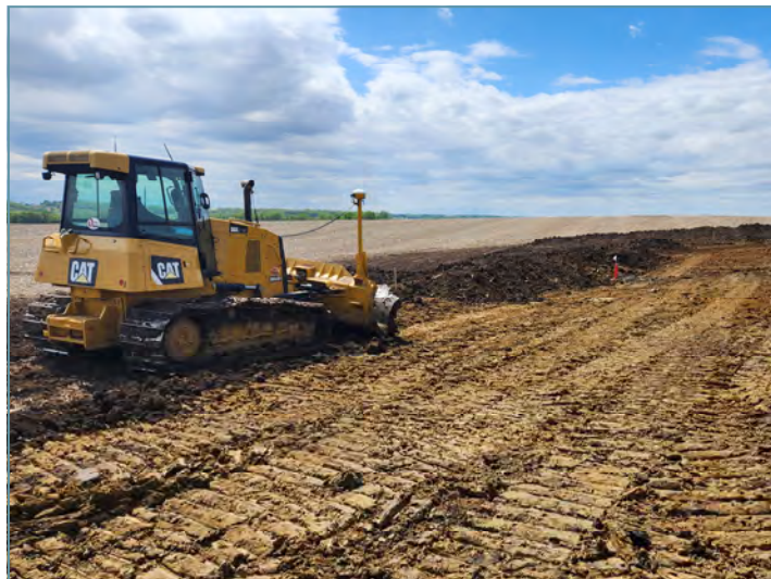
Topsoil was stripped back and stockpiled for later use.
