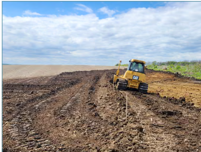
An earthen embankment was constructed to temporarily hold back runoff.
