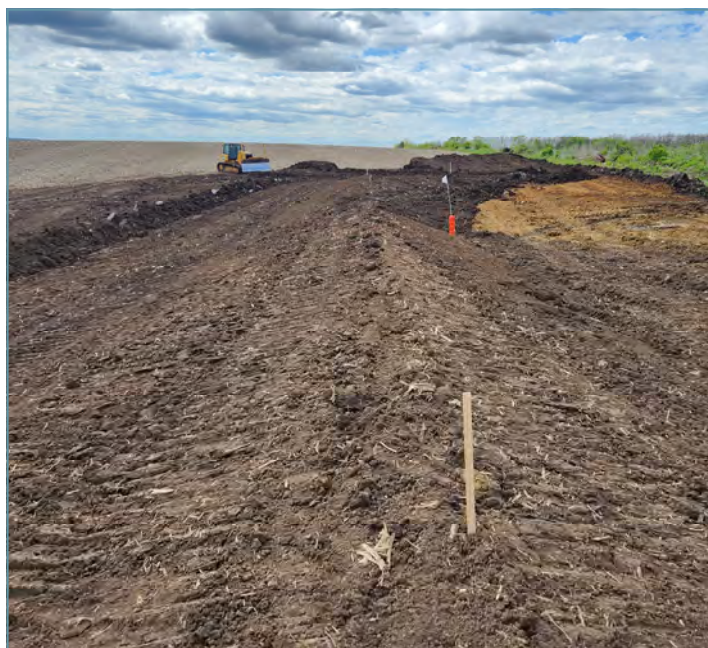
Topsoil was spread back over the site and the embankment was seeded with perennial vegetation.
