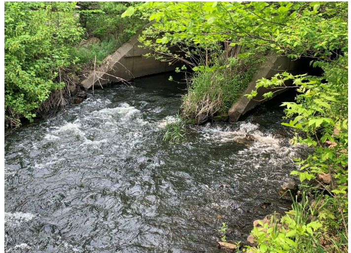
Figure 3. Downstream end of the culvert at the driveway crossing, which will be modified to deepen normal flow conditions.
